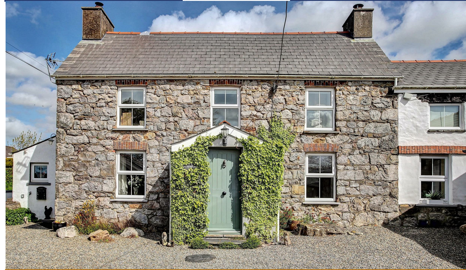
Upper Calf Field Camrose, Haverfordwest, Pembrokeshire, SA62 6HY
